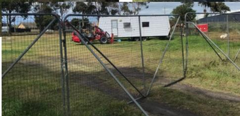
37 temporary fence panels with 2 trailers. Free standing, interlocking panels, 4.5m long x 2m high
